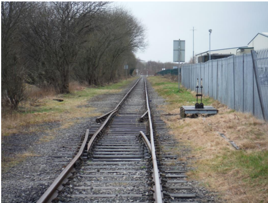
Network Rail / ELR boundary looking west (from Hopwood public footpath crossing)
