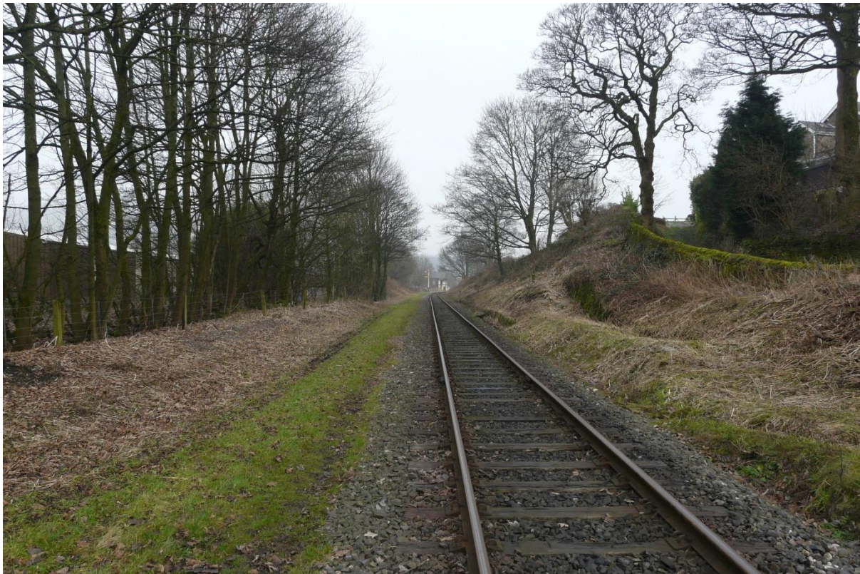
View North from Duckworth Lane crossing
