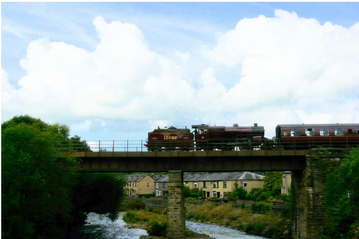
View West from 'waterside' pedestrian bridge
